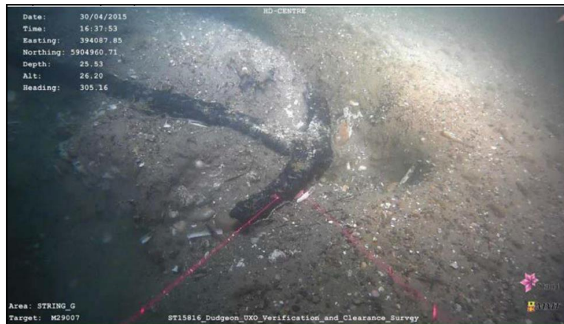
Figure 5: Debris showing scour formation (source Chapter 5 Project Description). 19
